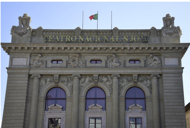
Fig. 8. Detail of the main facade of Teatro Nacional de S. João (1910–20) in Porto. (Photograph by authors).
