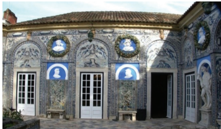
d. Music room exterior South wall.
