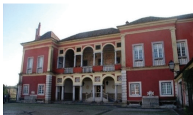
a. North Loggia façade – main entrance.
