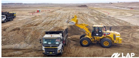
Appendix Figure 48: Construction progress at Lima airport
