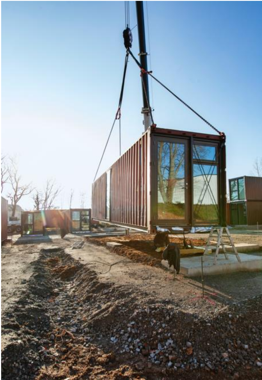
Figure 14: Strip foundations to avoid soil sealing
