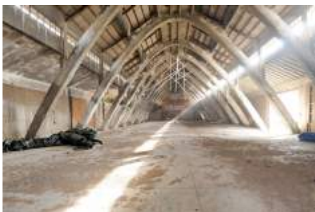
Fig.3 - Margherita di Savoia (BAT). Inside the warehouse designed and installed by P. L. Nervi (ph. A. Monte, 2007).
