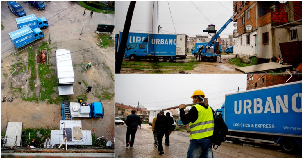
Figure 15. DEMOLITION OF BLOCK 10 (2018)
