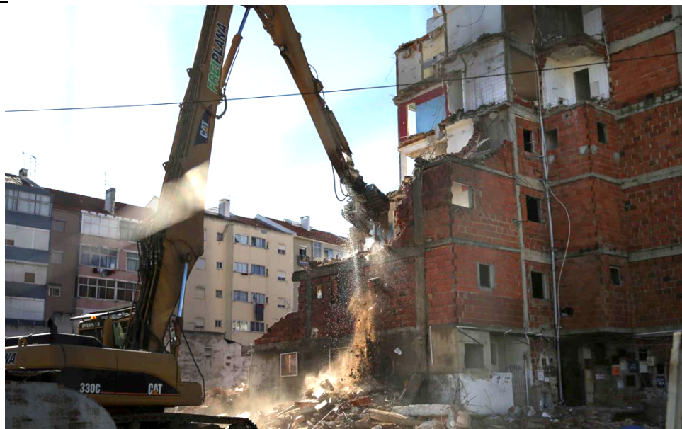
Figure 13. DEMOLITION OF BLOCK 10 (2019)
