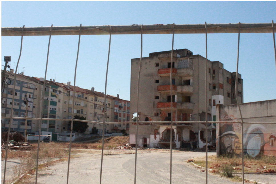
Figure 22. UNNUMBERED BUILDING IN THE DEMOLITION PROCESS (AUGUST 2023)
