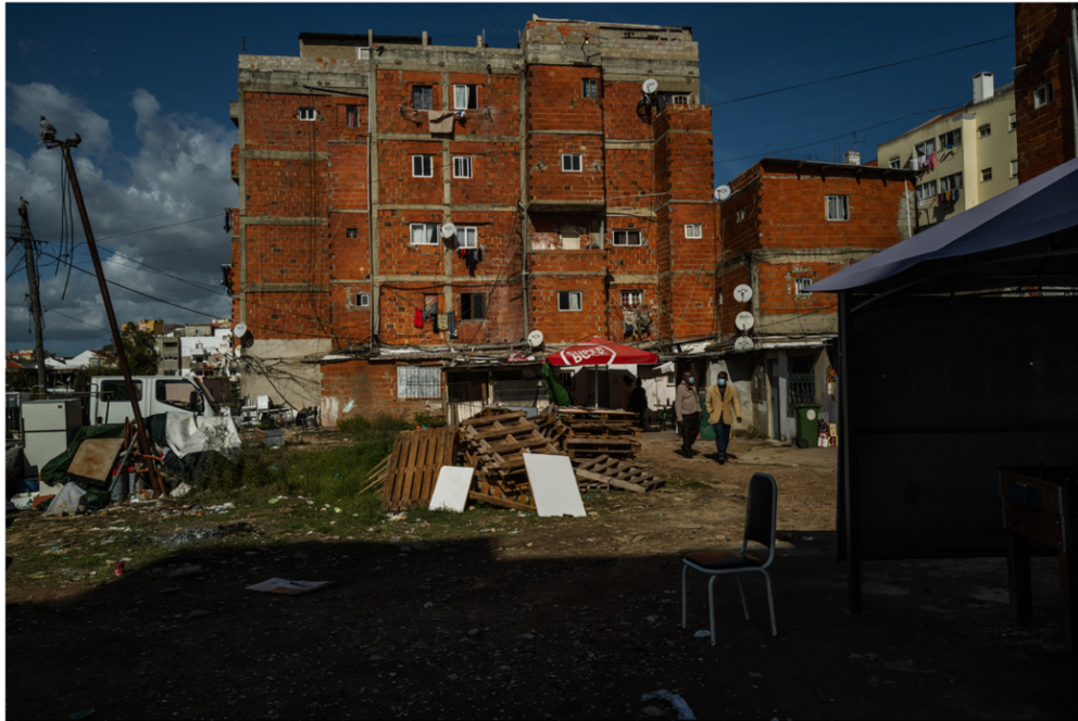
Figure 5. ONE OF JAMAICA’S BUILDINGS BEFORE DEMOLITION (2021)
