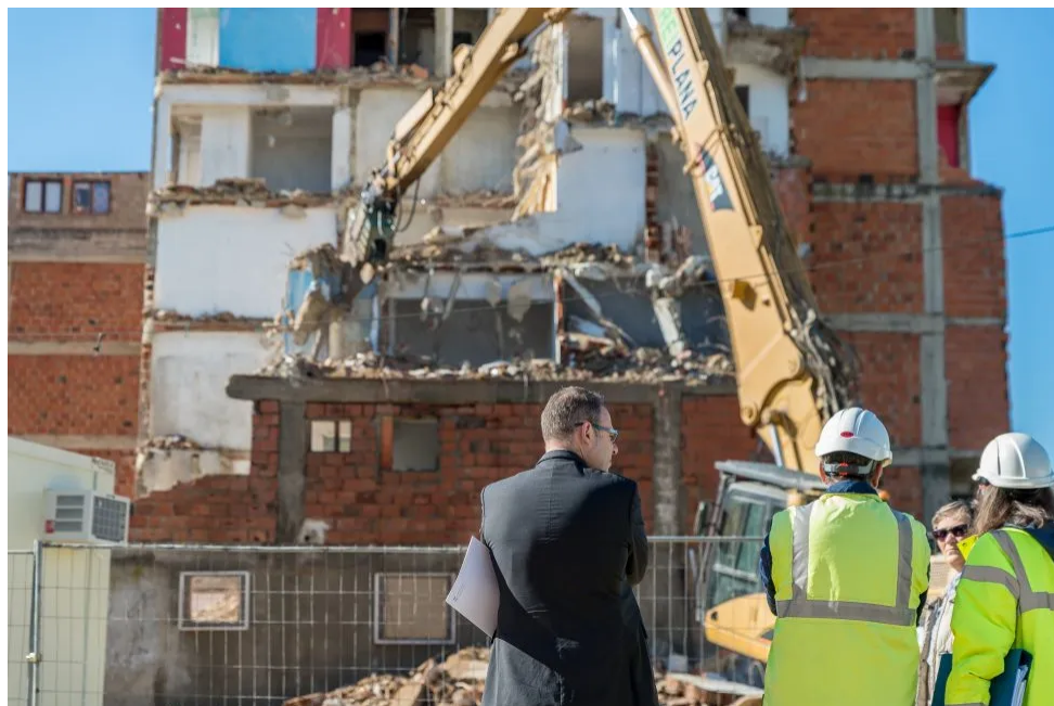
Figure 14. DEMOLITION OF BLOCK 10 (2019)
