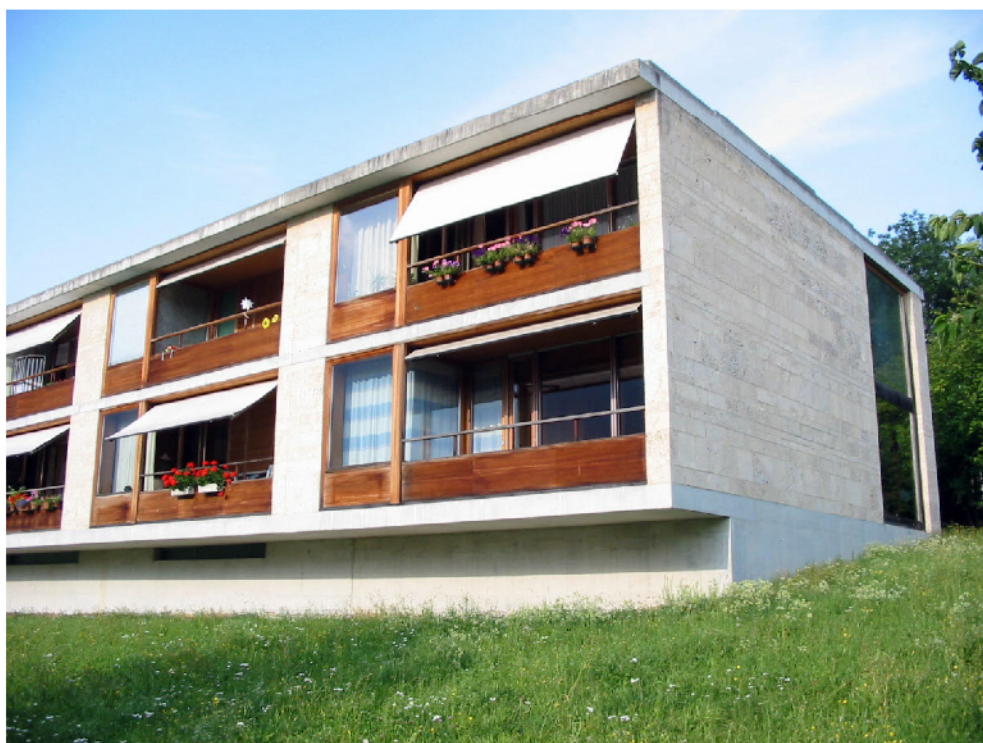
Figura 134 – Foto do exterior da Residential Home for the Elderly
