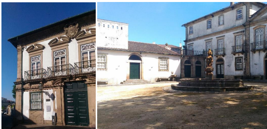
Figure 3. External facade (left) and internal facade(right) of the Biscainhos Museum .
