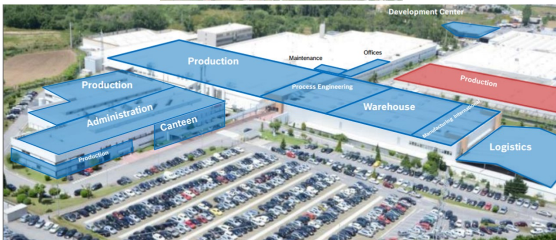
Figure 15 BrgP industrial plant. Adapted from the official presentation provided by BrgP.
