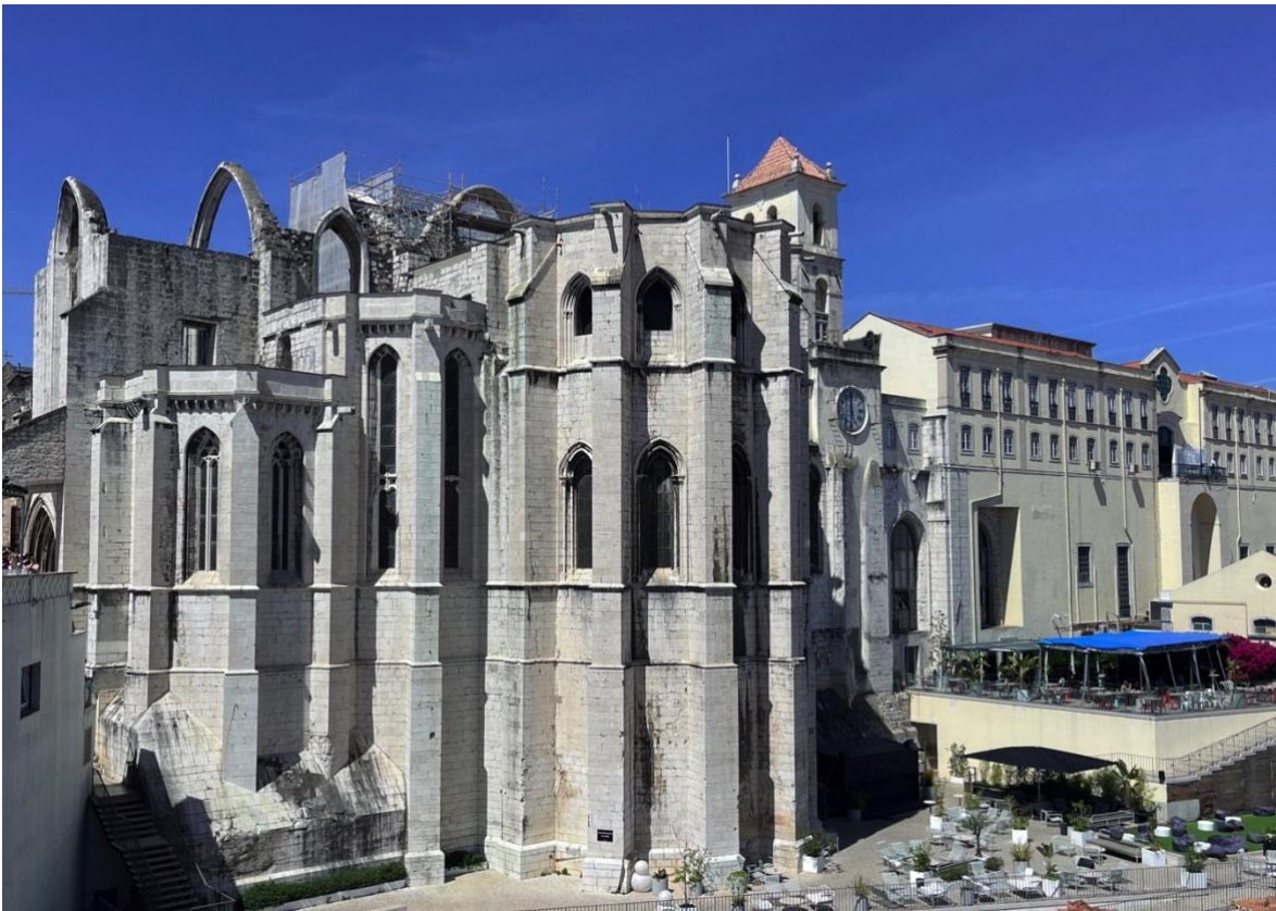
Figure 19 Convento do Carmo, view on the convent's roof, which collapsed during the earthquake in 1755, author's photograph (2023).
