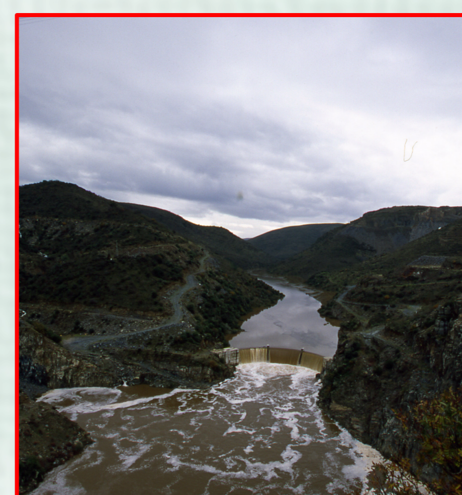
Embankment. Flooding in the 90s. Source: CNART photographic archive.
