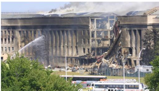
394262 07: Smoke comes out from the Southwest E-ring of the Pentagon building September 11, 2001 in Arlington, Va., after a plane crashed into the building and set off a huge explosion. (Photo by Alex Wong/Getty Images)
