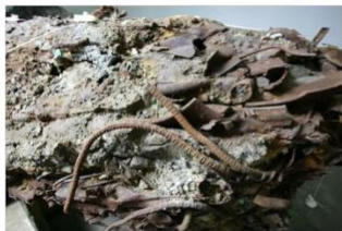
Four floors from the collapsed towers were compressed and fused into one mass. This is among the pieces of debris being stored at a hangar at Kennedy Airport, off limits to the public. James Estrin/The New York Times
