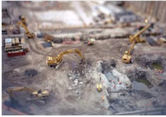
Construction in progress at ground zero on Aug. 16, 2006. This photograph was made with a tilt-shift lens on a Speed Graphic large format film camera, narrowing the field of focus. Fred. R. Conrad/The New York Times
