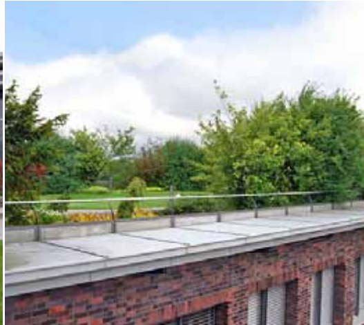
Sporty roof on an administration building in Brandenburg/Germany
