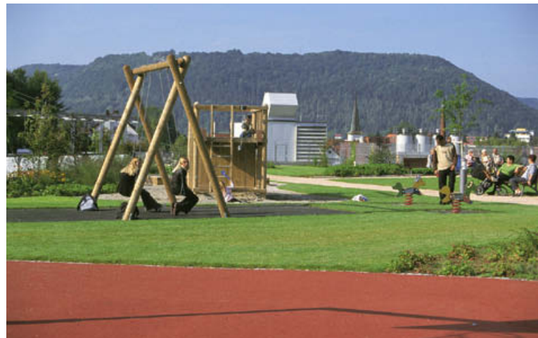
A prime example of community roof gardens – the public playground on top of a shopping centre in Geislingen/Germany. Copyright: ZinCo
