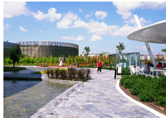
Oase of recreation on the Green Roof of Marmara Forum in Istanbul/Turkey
