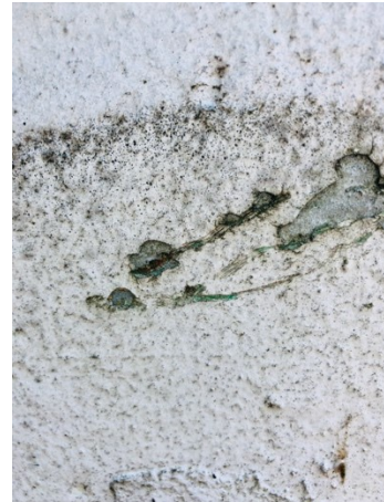
Fig. Att. 65 – Gap detail with active biological colonization in the white preparation layer.
