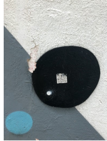
Fig. Att. 74 – Detail of detachment and vandalism with sticker in the chromatic layers.
