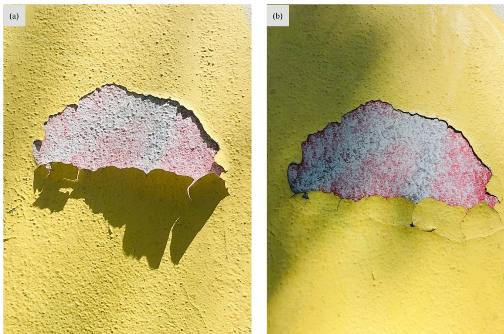
Fig. Att. 83 – Detachments in the upper right area of the work: a) before the intervention; b) adhesion with Plextol B500 with the original formula.
