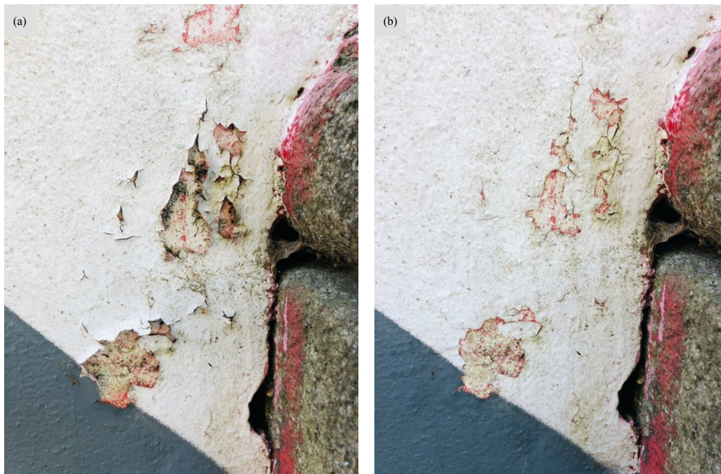
Fig. Att. 82 – Detachments in the lower right area of the work: a) before intervention; b) adhesion with Plextol B500 scattered at 15% in distilled water.
