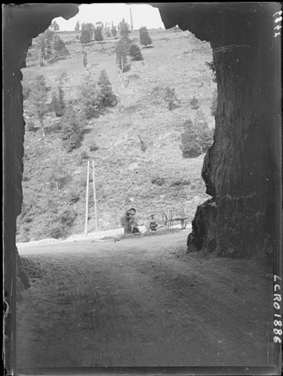
Tunnel de Kercabanac
