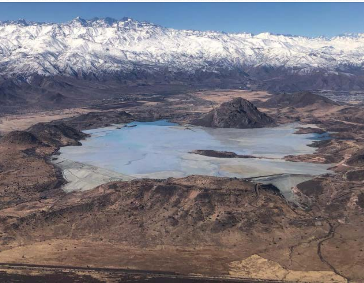
Fig. 2 - Las Tórtolas Tailings Dam of the Los Bronces Copper Mine Flotation Plant, Colina, Chile. [Digital Photograph] © Isidora Correa, 2024
