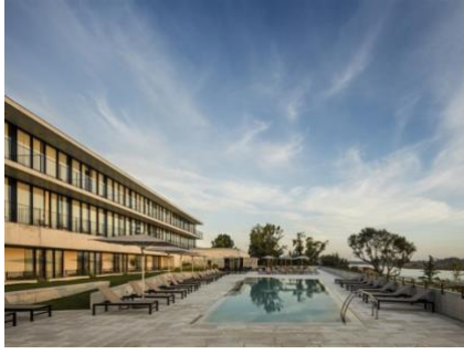
Figure 6: Montebelo Vista Alegre Ilavo Hotel, Portugal (Vista Alegre, 2023)
