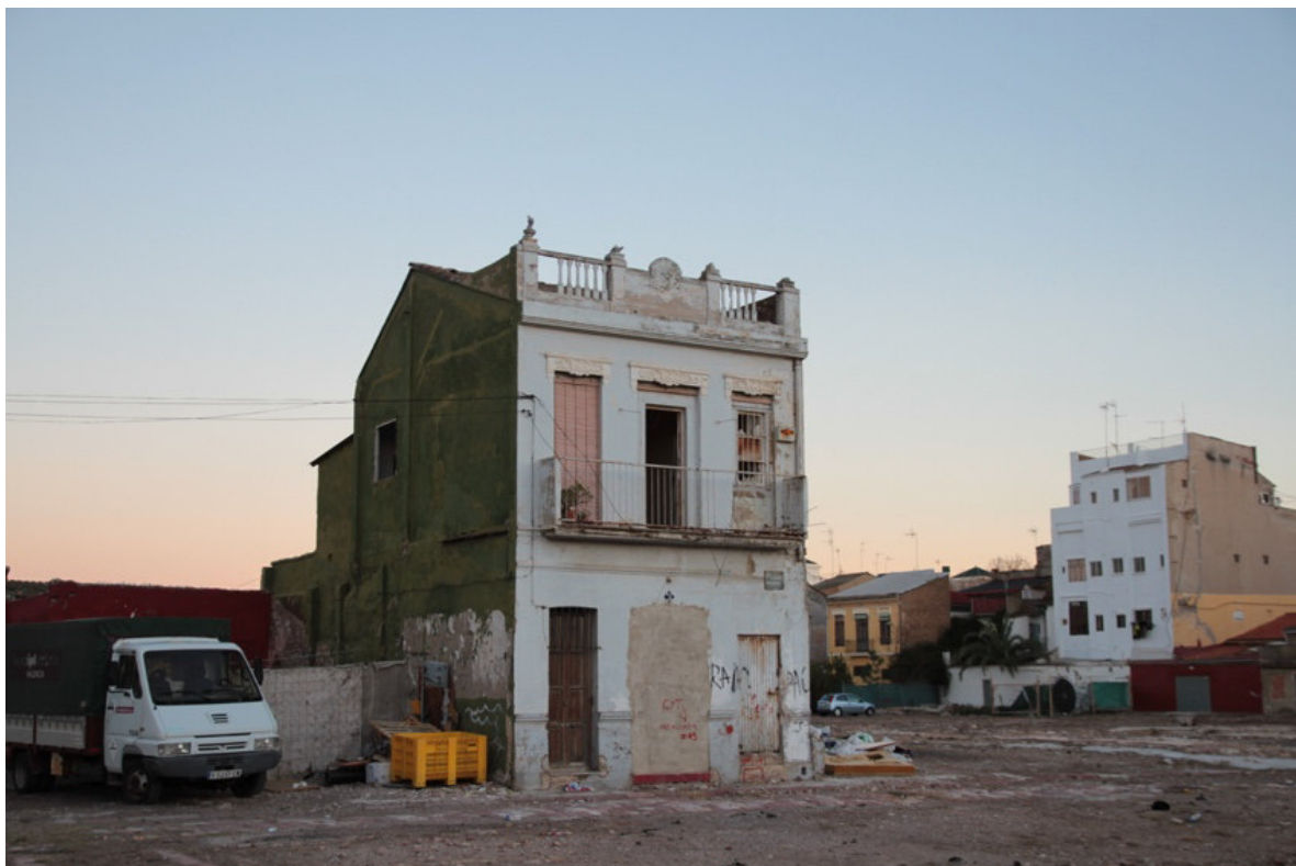
Fig. 15. El Cabanyal, Valencia. Partially demolished area.
