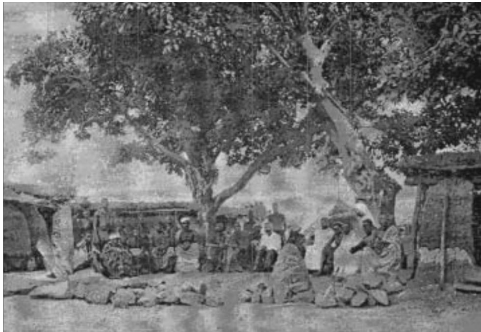
Figure 7. Picture of ‘The Village Street in Akpafu’, from The Ewe People: A Study of the Ewe People in German Togo , Jakob Spieth 2011 (1906): “Houses are usually clustered together along a wide village street, with a big shade tree in the middle. This is the center where the villagers have their entertainment, meetings, and games” (34).
