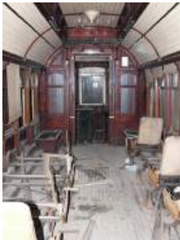
Fig. 5 - Current condition of the tram's interior.
