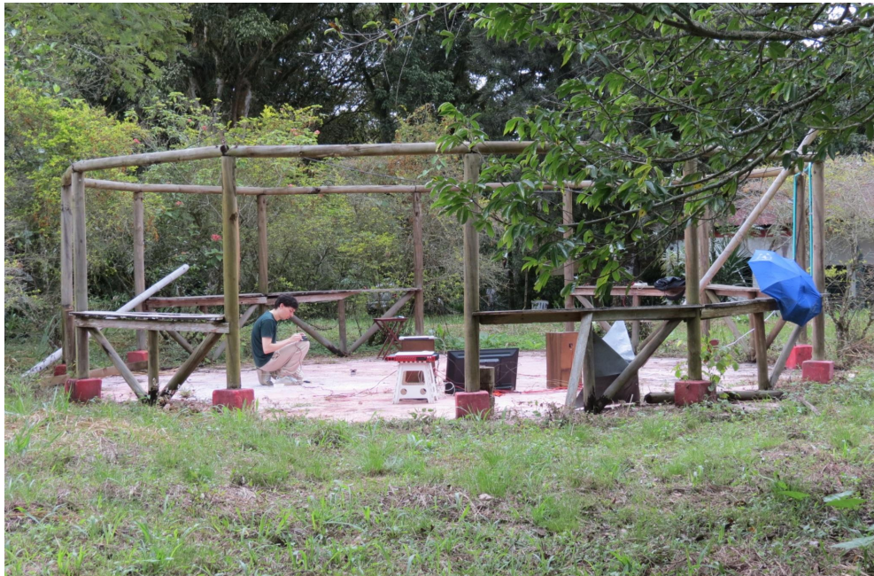
fig 31. view of the on-site sound installation. source: figure produced by the author.
