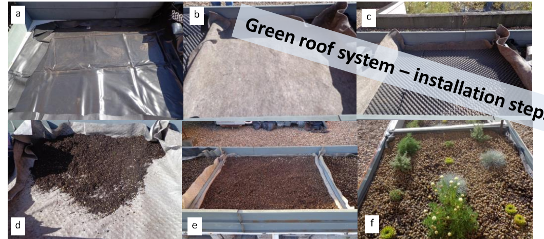
a- impermeabilization membrane; b- geotextile membrane (470 g/m 2 ); c- drainage layer; d- geotextile membrane (150 g/m 2 ); e- substrate mixture; f- vegetation
